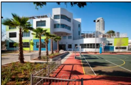
Figure 4.4 – Elementary school in Tel Aviv. Source: (Jackobson, 2017)
