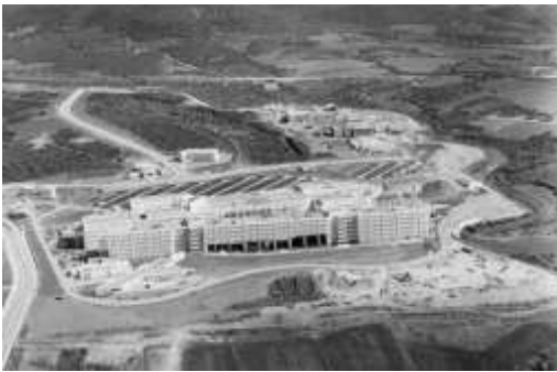
Figure 1. General view of the Hospital of Alexandroupoli (aero photography).
