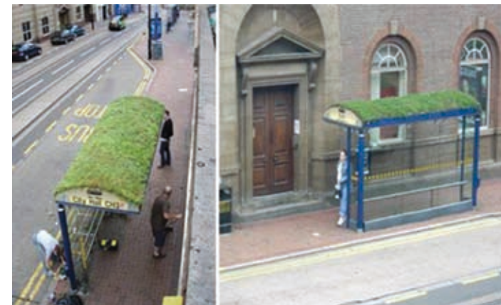
Bus Shelters. West Street – Sheffield
