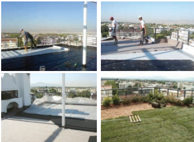
Picture 10. Step by step installation of an intensive greenroof in Attica
