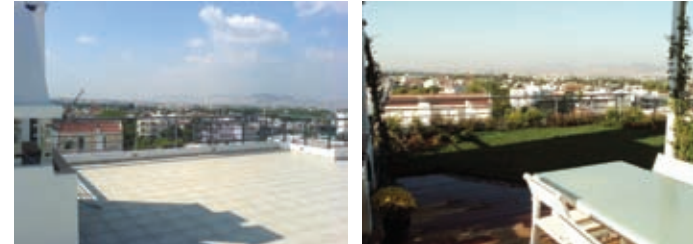
Picture 11. Before and after the construction of the greenroof
