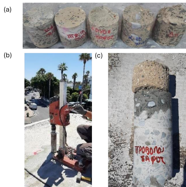
Figure 3: (a) Concrete core sample; (b) Extraction of core sample and (c) Cantilever's core sample (Durable Engine Structural Engineering LLC Archive).
