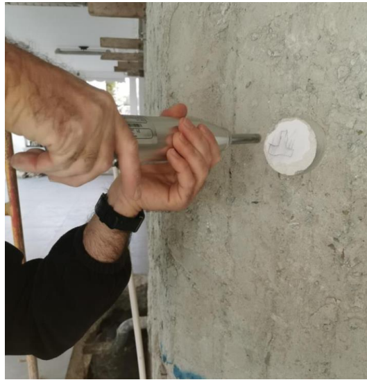
Figure 4: Non-destructive testing of concrete employing Schmidt Hammer.
