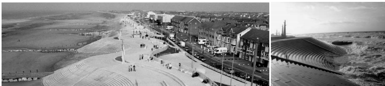
Figures 10, 11: The coastal front after the completion of the project
